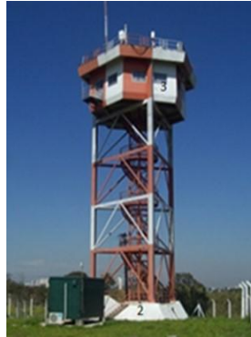
Fig. 1–Outdoor view of tower where the gamma ray detector are installed.
